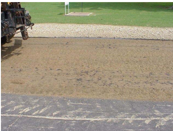
(5) Sand Applied Prior to Scrubbing
