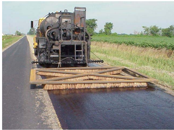
(2) Scrubbing the Oil into the Roadway
