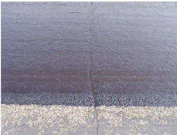
(3) Oil Penetrates and Seals Cracks
