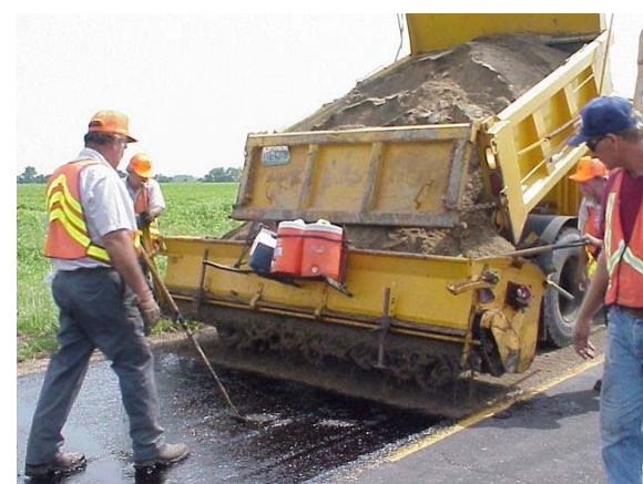
(4) Applying the Sand
