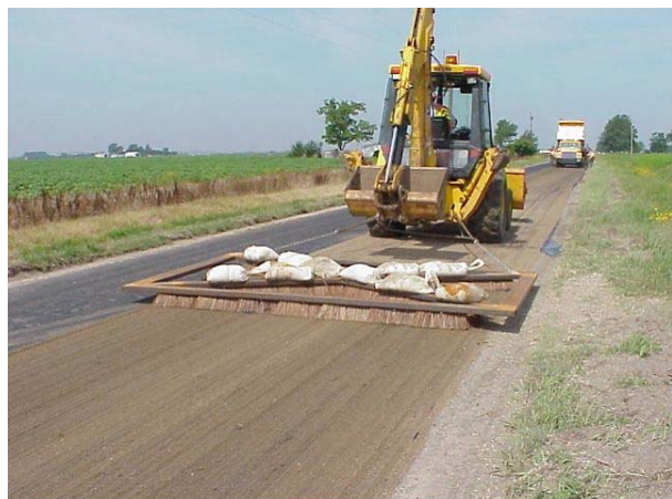
(6) Scrubbing the Sand
