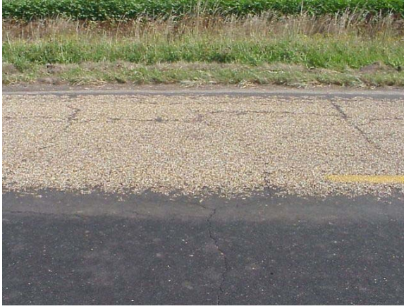
(1) Roadway Prior to Scrub Seal
