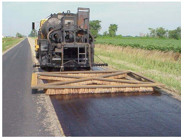
(2) Scrubbing the Oil into the Roadway
