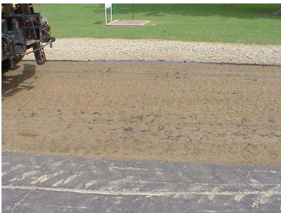
(5) Sand Applied Prior to Scrubbing
