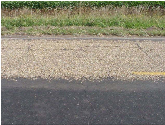
(1) Roadway Prior to Scrub Seal
