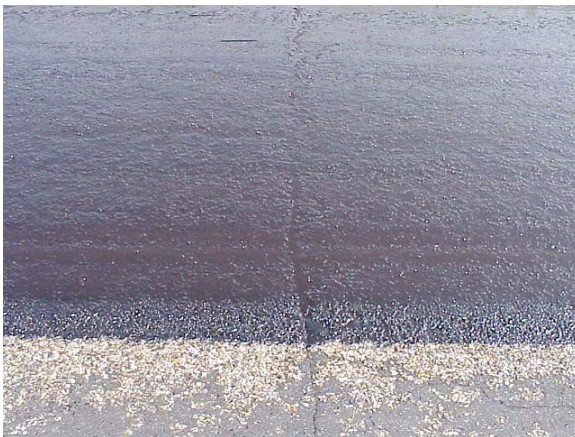
(3) Oil Penetrates and Seals Cracks
