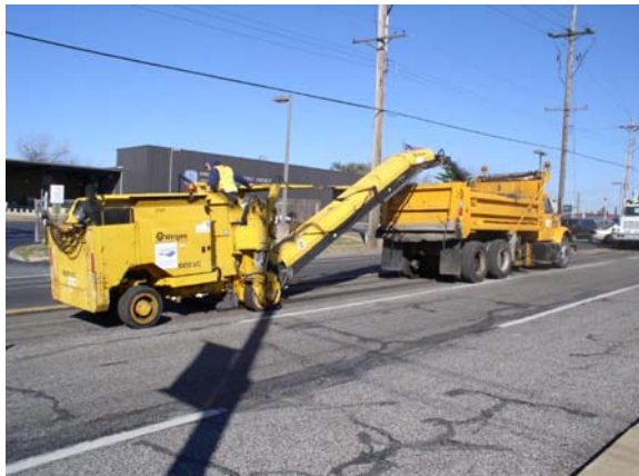
(1) Pavt Repair Milling Operation
