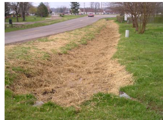
(6) Mulched & Seeded Ditch – Finished Product
