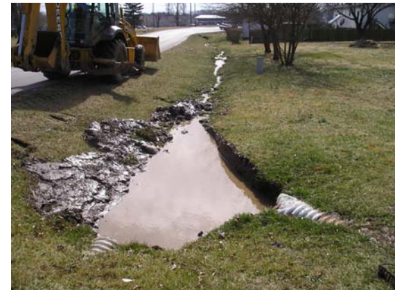
(4) Digging out Culvert Ditch
