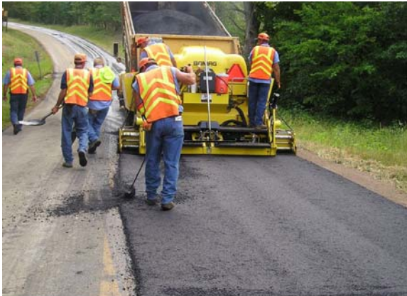
(3) Hand Raking as needed
