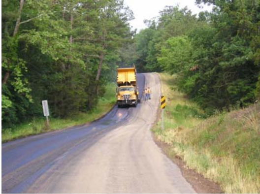
(1) Asphalt Pavement Repair
