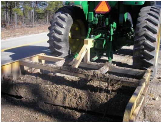
(1) Pulling Shoulders with a Grademaster
