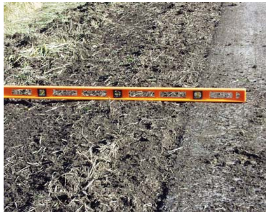
(6) Shoulder Reclamation - Final Product
