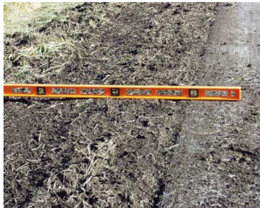
(6) Shoulder Reclamation - Final Product
