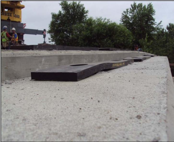
Cap finish on skewed bridges should follow the grades established in the contract drawings (see Figures 3 and 4). This should provide a smooth surface though not necessarily a straight edged surface. Cap concrete on skewed bents should be finished parallel to the roadway.
