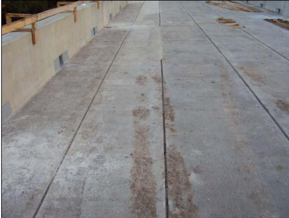
Figure 10 - All Three Differential Camber Conditions Present
