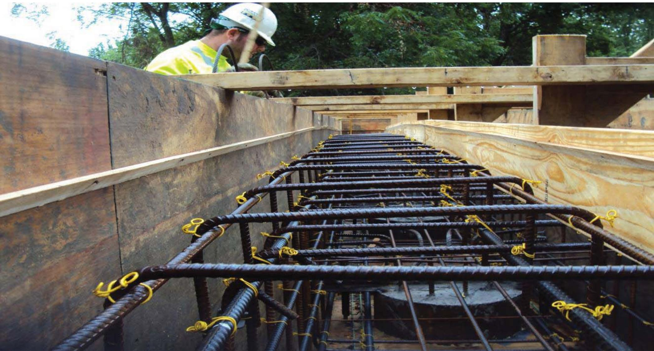
**APPENDIX 13 – BEAM CAP BEARING AREA BEING CHECKED WITH STRAIGHT EDGE**
