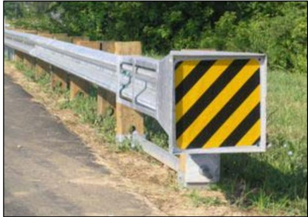
Figure 18 - Guardrail End Terminal
