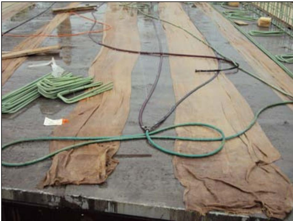
Figure 11 - Good Grout Curing
