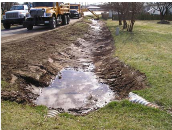
(5) Graded Culvert Ditch
