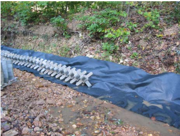
(5) Ajax Installation with Silt Blanket
