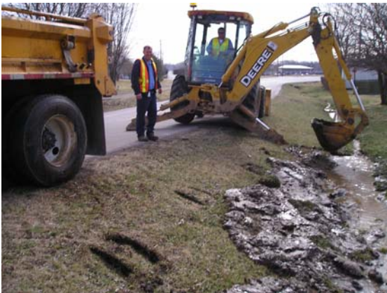
(3) Digging out Culvert Ditch
