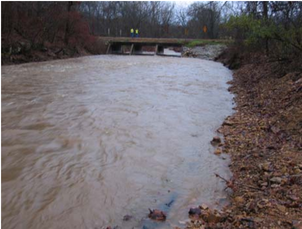
(3) Indian Creek – Upstream of Triple Box Culvert at Route AM
