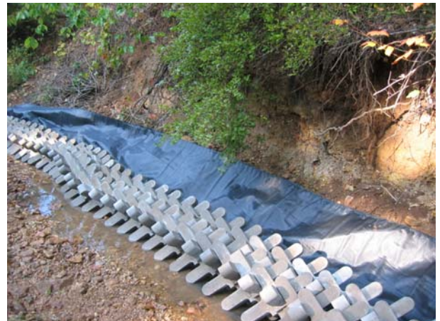
(6) Ajax Installation - Continued
