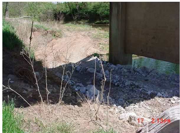
(10) Preliminary Grading for Gabions
