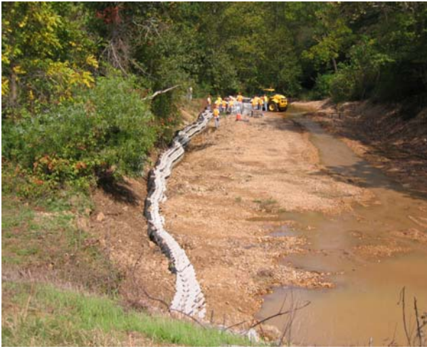
(7) Completed Installation of Ajax Blocks
