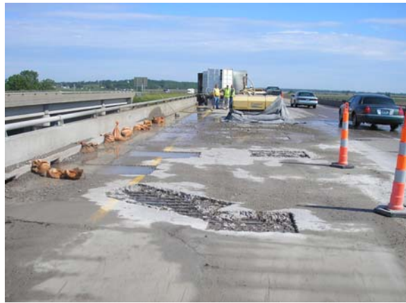
(4) Results of Hydro demolition for Spot Patching
