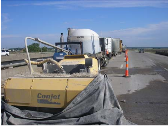
(1) Hydro Demolition Set Up for Spot Repair
