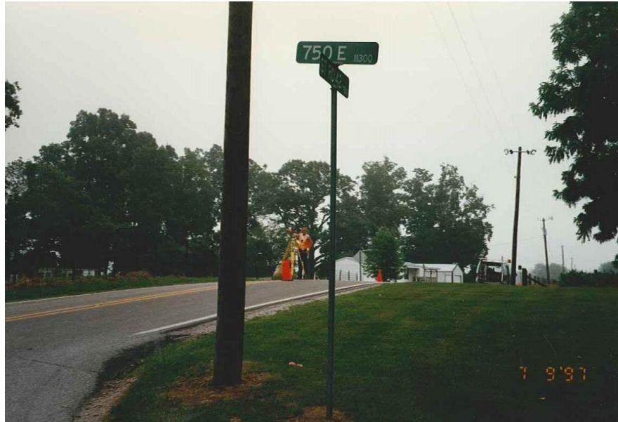
Figure 6.2 Intersection sight distance obstructed by hill.
